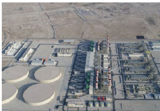
Umm Al Houl Power Project / Qatar Capacity : 2,520MW (504MW), 198MIGD (39.6MIGD) / Gas fired & Water produce Share : 20% Partners: QEWC, QatarEnergy, Qatar Foundation, JERA
