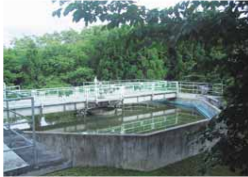
Water treatment facility
