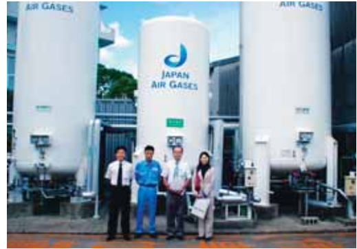
Onsite inspection of industrial gas management
