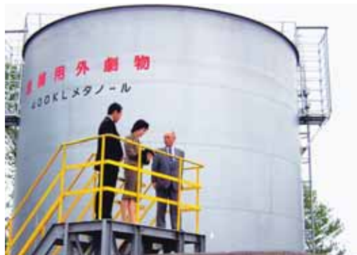
Onsite inspection of methanol safeguarding management structure
