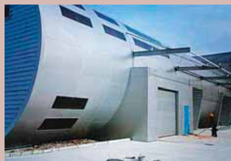
Shanghai MegaThin ® plant
