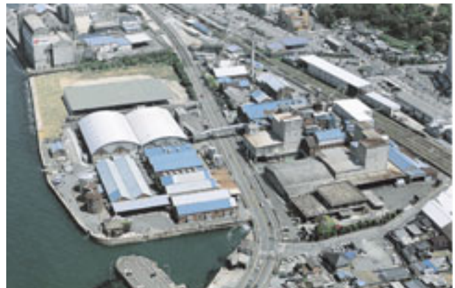
Boiler fuel conversion at Kanmon Seito leads to reduced CO 2 emissions
