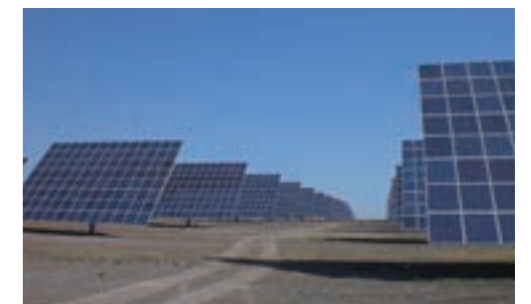
The solar photovoltaic project in Moura, Portugal
