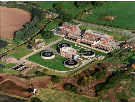
Seedy Mill Treatment Works
