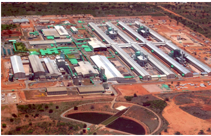
Aerial view of the Mozal aluminum smelting facility
