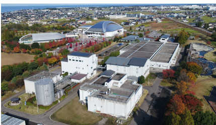
Kurobe City Sewerage Biomass Energy Reuse Facility
