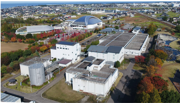
Kurobe City Sewerage Biomass Energy Reuse Facility
