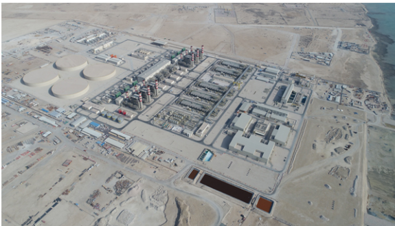
Umm Al Houl Power, Qatar
