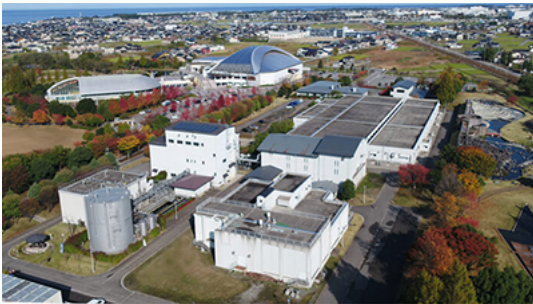
Kurobe City Sewerage Biomass Energy Reuse Facility
