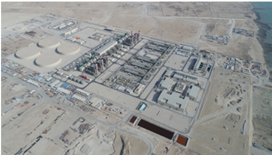
Umm Al Houl Power, Qatar
