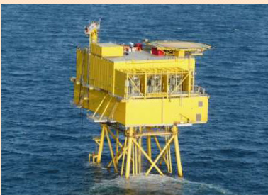
Offshore substation in the U.K.
