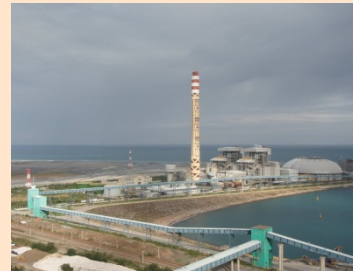
Coal-fired power station in Taiwan
