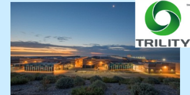
Desalination Plant in Adelaide
