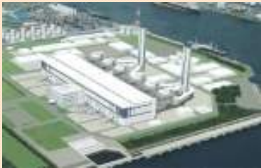
Gas combined-cycle power station
