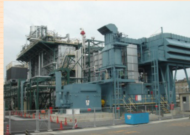
Gas turbine power station near Nagoya
