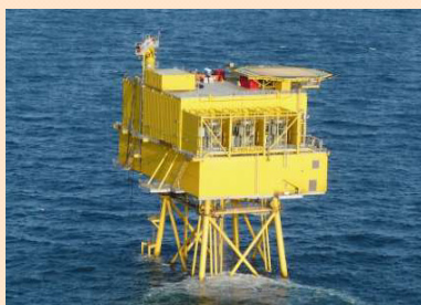
Offshore substation in the U.K.
