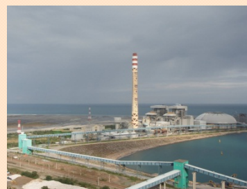
Coal-fired power station in Taiwan
