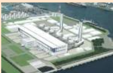
Gas combined-cycle power station
