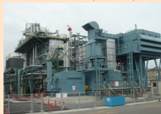
Gas turbine power station near Nagoya
