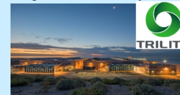
Desalination Plant in Adelaide
