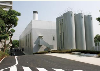
Energy Center at the Isehara Campus of Tokai University
