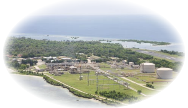
View of gas processing plant (Pangerungan Island)
