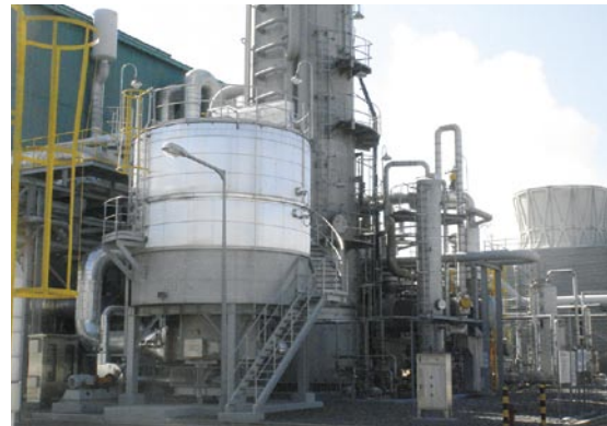
An N 2 O removal facility
