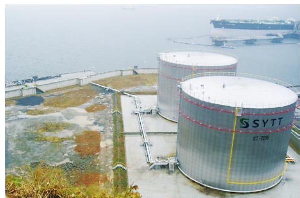
Tanks built by MCK in Yeosu
