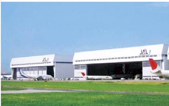
Haneda Airport Maintenance Center (IIF), an industrial REIT property
