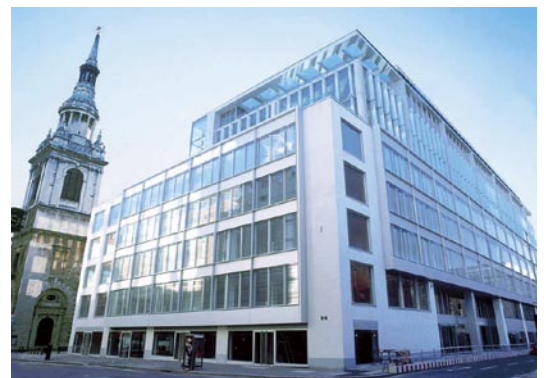
MC was involved in developing Bow Bells House, a building combining office and commercial retail space in the City of London.
