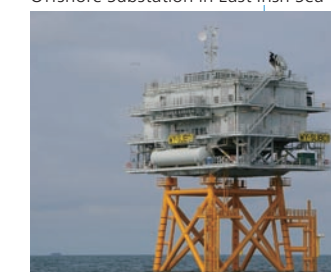
Offshore Substation in East Irish Sea
