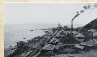
The Takashima Coal Mine
