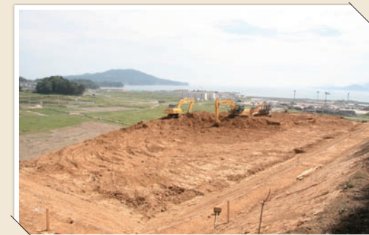
▲ Land is being readied for reconstructing the hotel.
