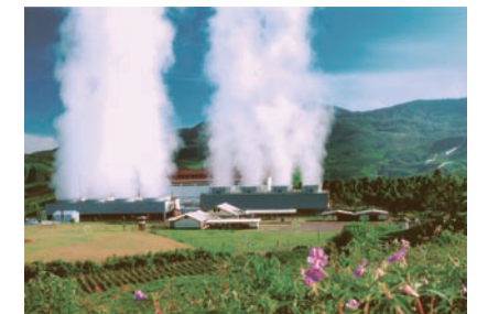
Wayang Windu Geothermal Power Project Plant
