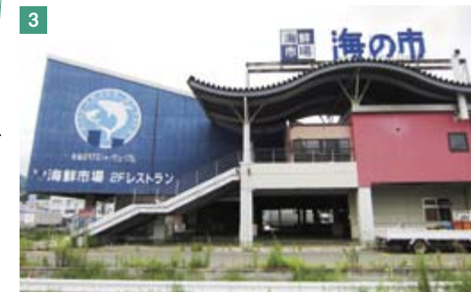
Supporting the "Umi no Ichi" seafood market adjoining the Kesenuma fish market. In addition to providing employment for around 10 people, the market will offer employment opportunities at tenant companies; before the disaster tenants provided jobs for about 120 people.
