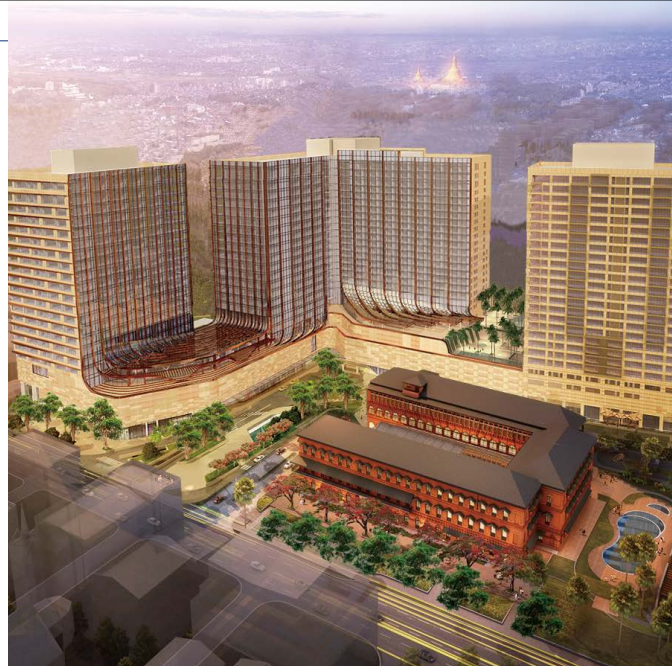
Image of completed "Landmark Project" (Yangon)
