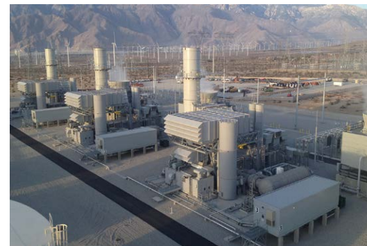
Sentinel Power Plant owned by DGC (California, U.S.)
