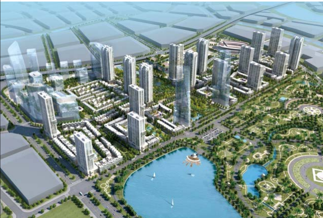
Image of completed "TMCP Project" (Hanoi)
