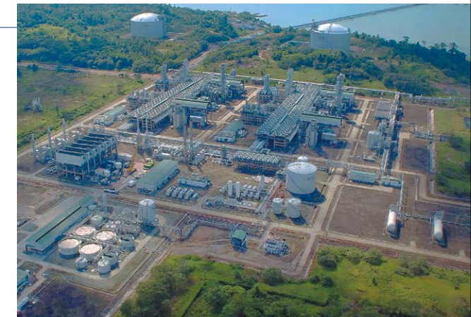
Existing LNG process trains, tanks, and jetty (The expansion work is scheduled to start in the third quarter of 2016)
