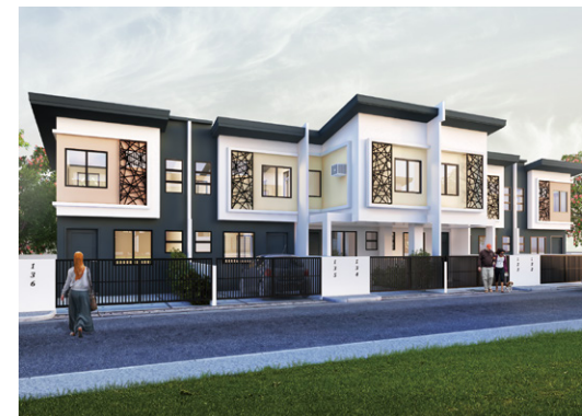
Image of some residential houses
