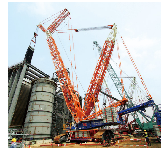
Mobile crane at work
