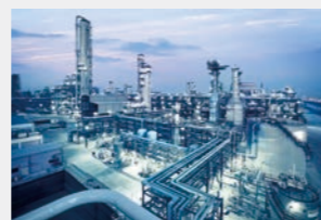
Saudi Petrochemical Project
