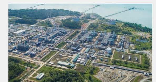
Liquefaction plant existing second system and expanded system under construction, LNG tanks, jetty, etc.
