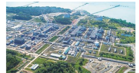
Two existing LNG trains and an expanded train under construction, LNG tanks, jetty, etc.
