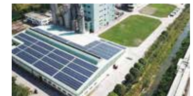
Thai Shinkong Industry Corporation Ltd. (TSIC) PET manufacturing plant, which increased capital in 2020 (See page 99 for information on the Chemical Recycling Business)
