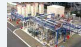
Dehydrogenation plant in Kawasaki City
