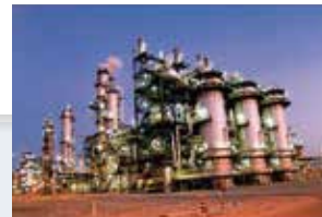
Saudi Petrochemical Project
