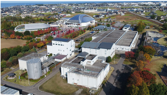
Kurobe City Sewerage Biomass Energy Reuse Facility
