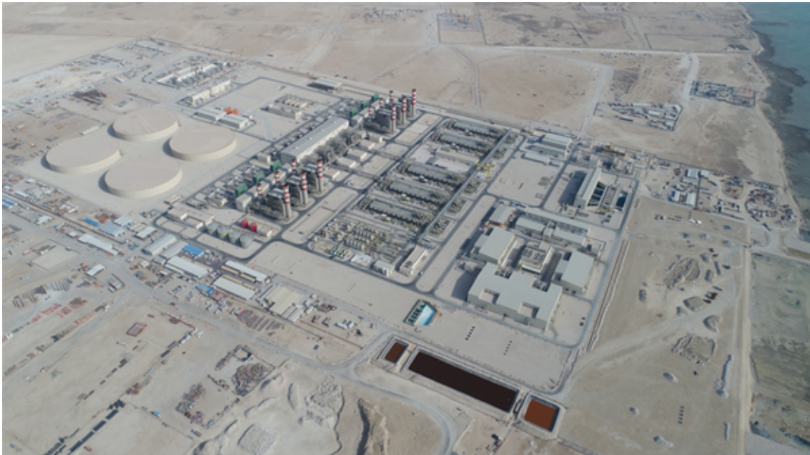
Umm Al Houl Power, Qatar
