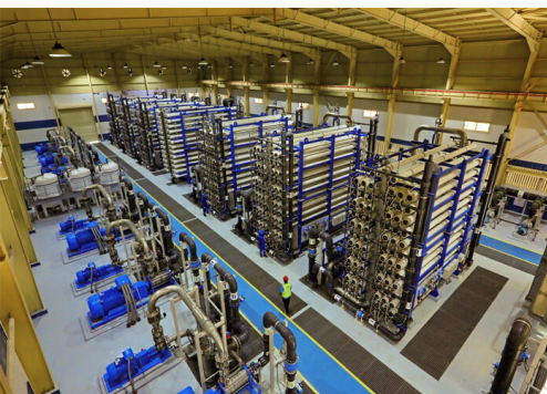
Al Yosr Desalination Facility, Egypt
