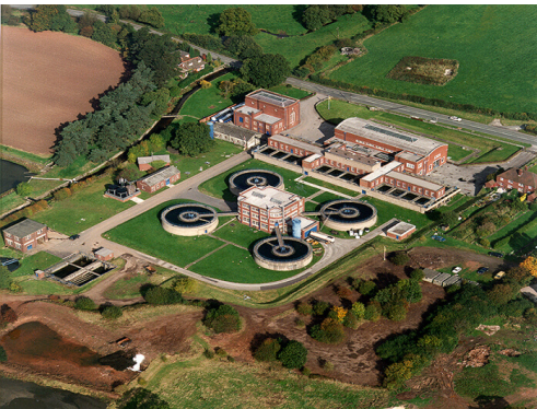
Seedy Mill Treatment Works
