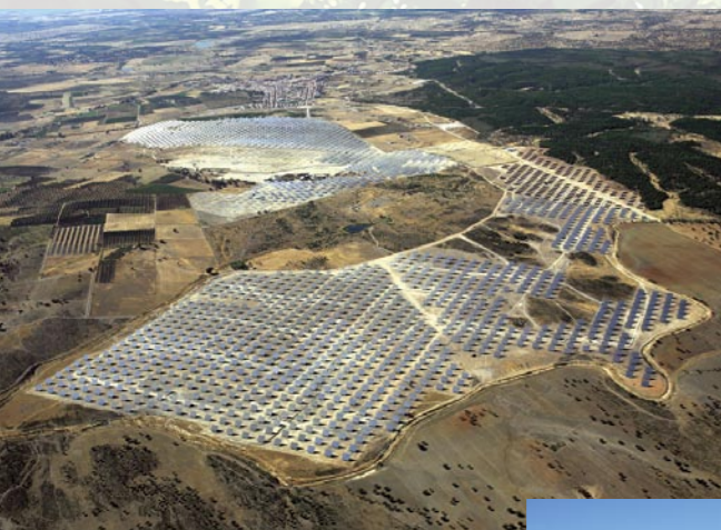
Power station in Moura, Portugal Around 260,000 solar cell panels are laid out over an approximately 250 hectare site.
