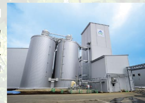
Hokkaido Bio Ethanol's plant in Shimizu town, Hokkaido prefecture commenced operations in March 2009. This new facility is expected to produce 15,000 kiloliters of bioethanol per year.
