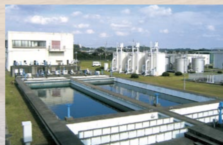
With this waterworks project along the Nagatogawa river in Chiba Prefecture, Japan Water Corporation became Japan's first company to sign a combined DBO (Design, Build, Operate) contract.
