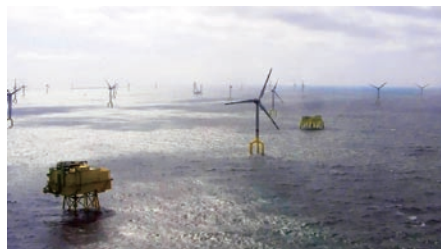
Offshore transmission cables and related transformers are being constructed in the German North Sea.
