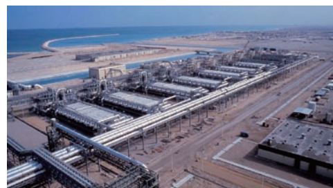
Seawater desalination plant
