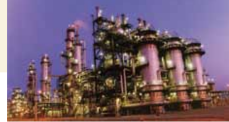
Saudi Petrochemical Project (Saudi Arabia)
