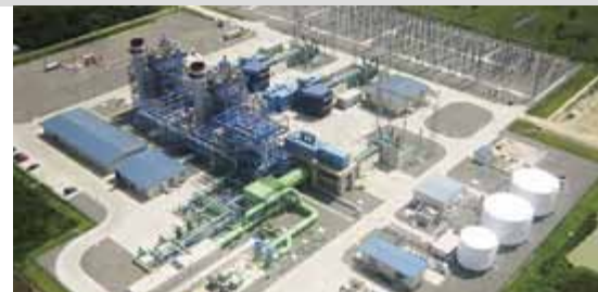
Tuxpan V Power Plant
