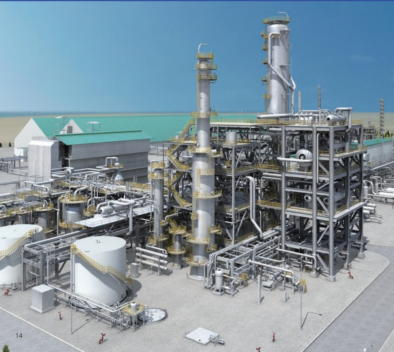
Turkmenistan P16 Large-scale Fertilizer Plant Project
