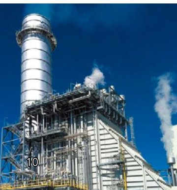
■ Navoi combined cycle power in Uzbekistan, an MC/CE joint project
