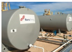
■ Crude oil production site
