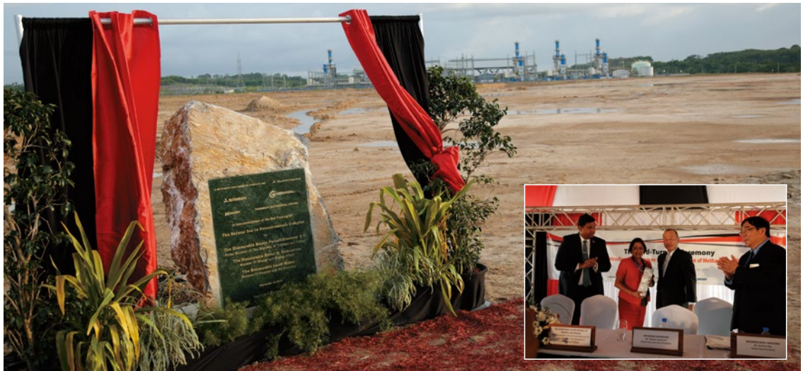
■ Planned plant construction site / Groundbreaking ceremony
