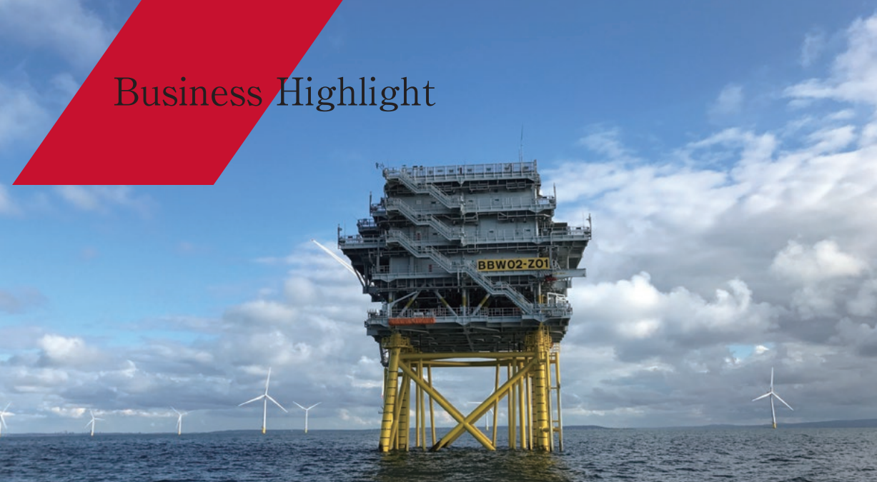
Offshore wind substation
