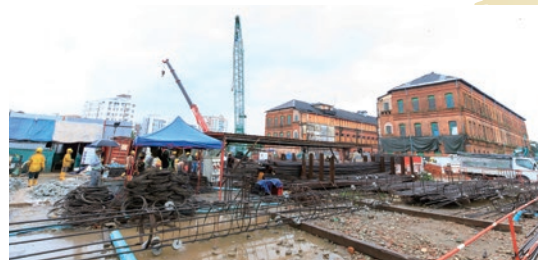
As Yangon experiences a long rainy season, work interruption due to downpours happens almost daily. Despite such bad conditions, the construction is progressing safely and on schedule based on the plans
